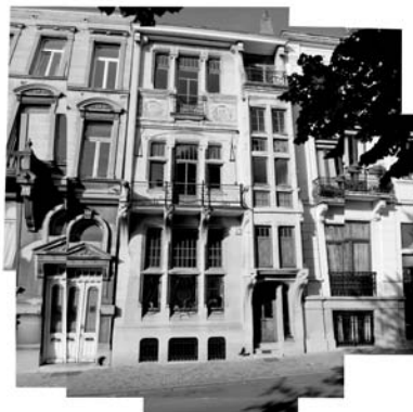
place Moricharplein 41, 1900 arch. E. Blérot
